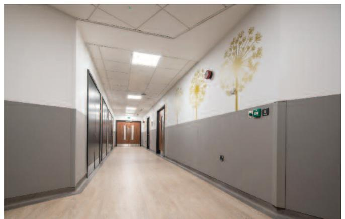
Sheet wall protection can be cut into bespoke designs.
